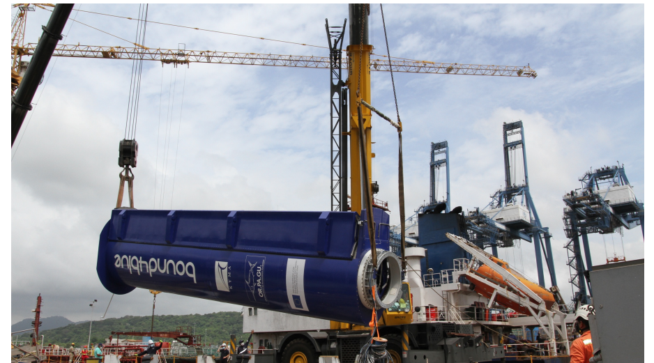
First 12-meter eSAIL® unit being installed at the shipyard (Panama)
