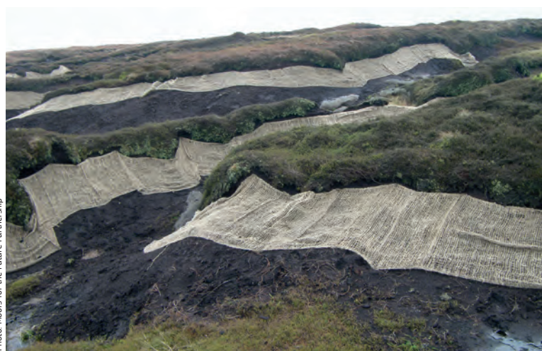
These geotextiles protected bare peat from erosion and provided a stable base for plants to grow
