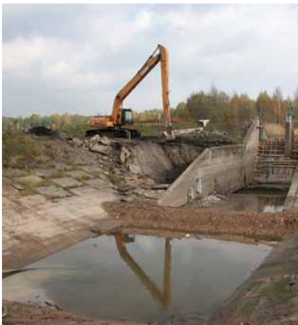
Reconstruction of Žuvintas sluice
