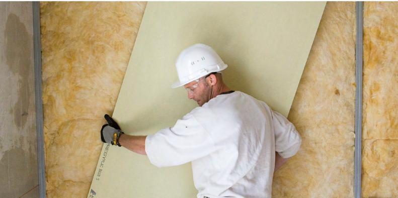
The Gypsum to Gypsum project has manufactured new drywall from 30% recycled material.
