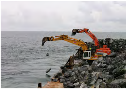
Placement of boulders
