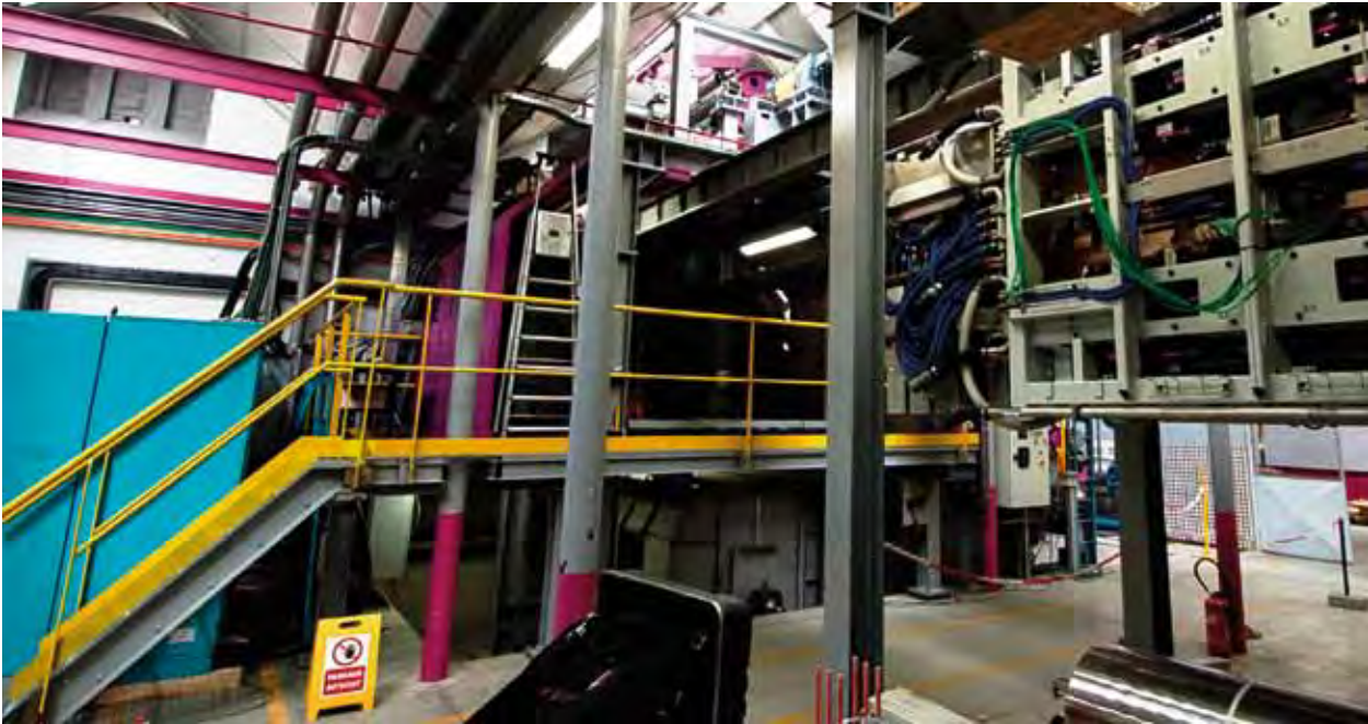
A 20% substitution of current stainless steel processing lines with the ECOTRANSFLUX technology would significantly reduce nitric acid and hydrofluoric acid consumption
