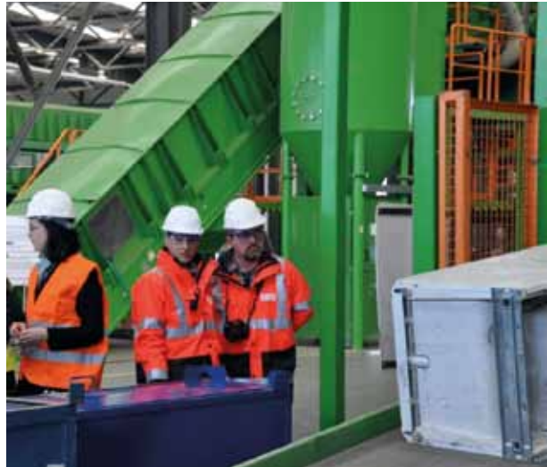
An audit being carried out in the “Green WEEE” plant in Buzau in Romania
