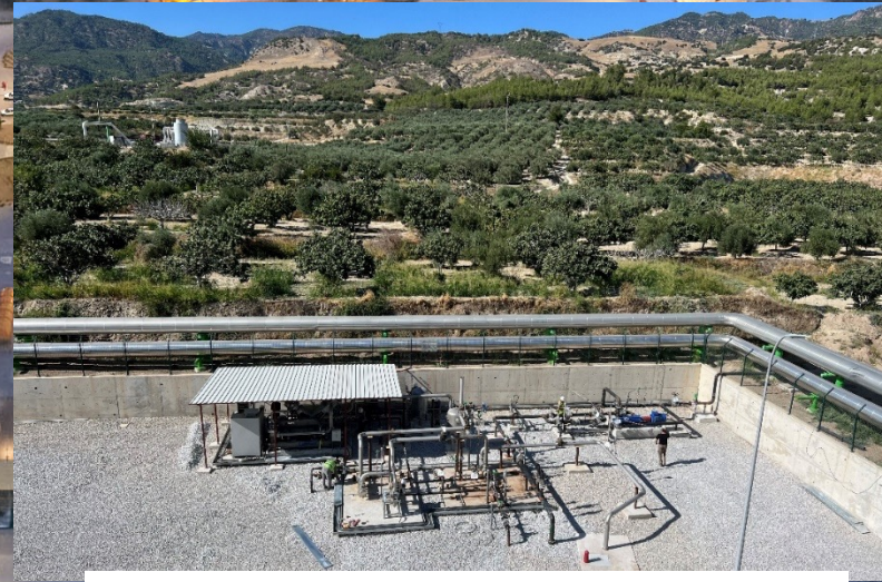
NCG capture and injection system - ZORLU
