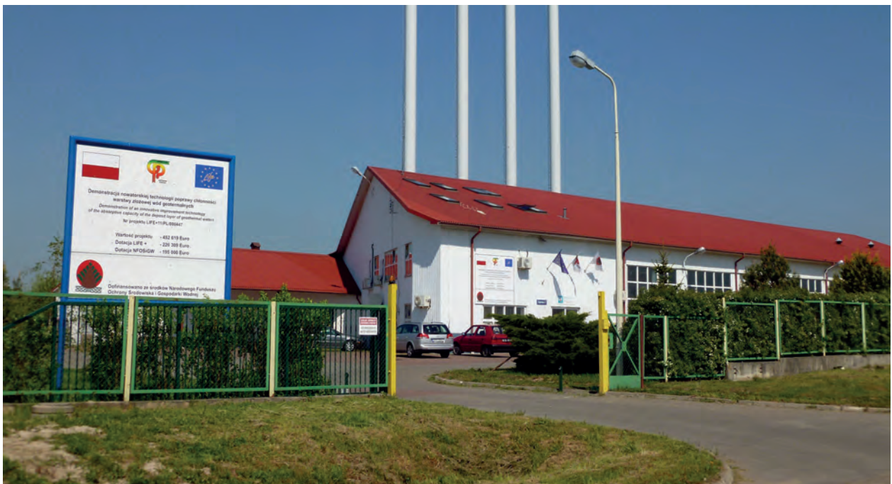
The project was implemented in the geothermal plant of Pyrzyce, Poland
