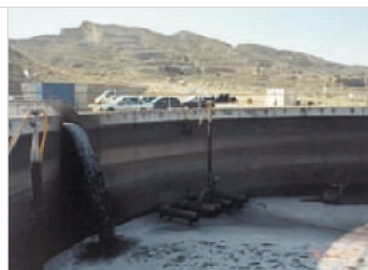
Biological reactor for continuous treatment of the wastewater.
