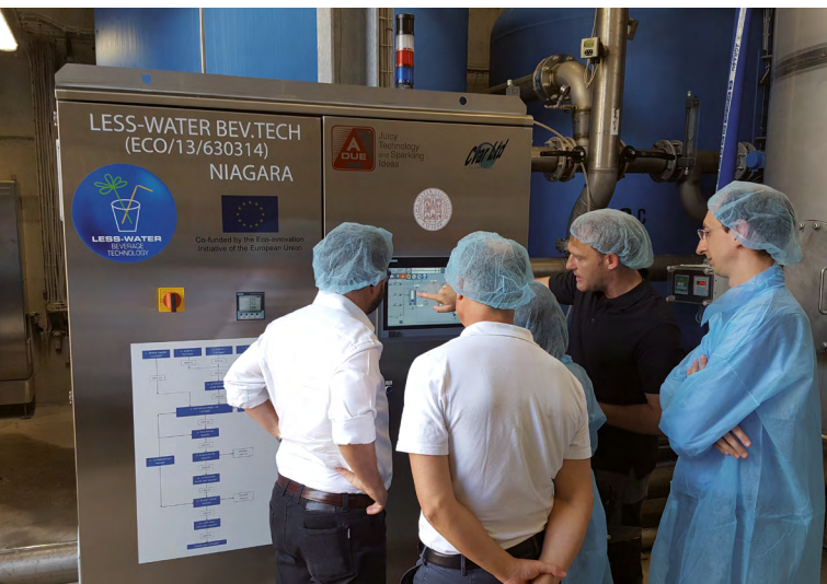
Reverse osmosis water treatment system
