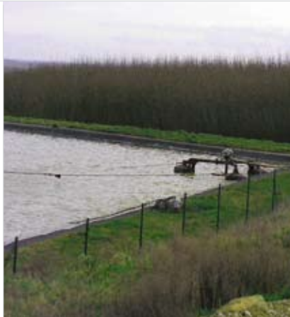
The purifying properties of willow coppice on sewage sludge reduced nitrates and phosphorous below levels required by European legislation on urban residual water
