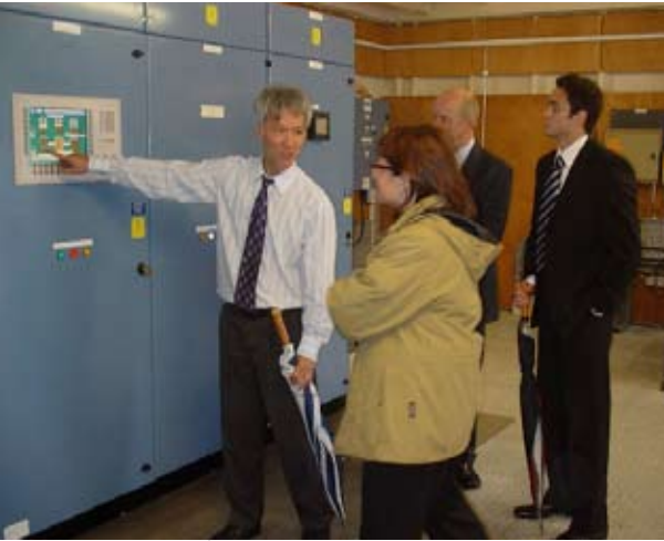
Son Le from United Utilities demonstrates the six small vessels in series that allow greater control of the reaction conditions and therefore greater gas production.
