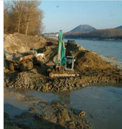
Removal of the artificial river banks restored natural erosion and improved the floodplain habitats
