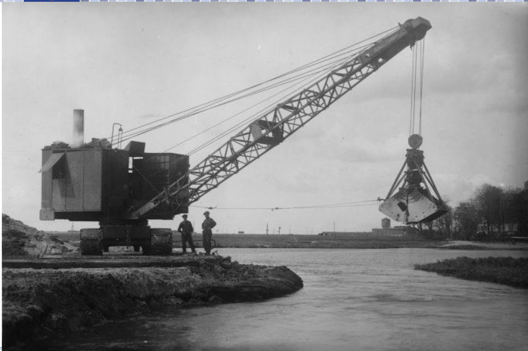
Drainage work of the Tønder marsh 1927
