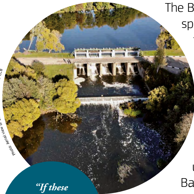
Photo: the Stracha River Dam © CCB
