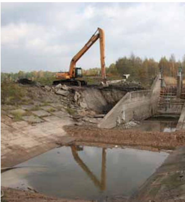
Reconstruction of Žuvintas sluice
