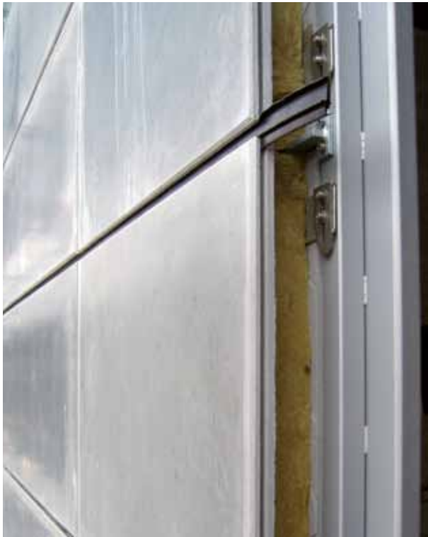
The basic element of construction is made of two shells of textile reinforced concrete combined with rigid polyurethane foam insulation
