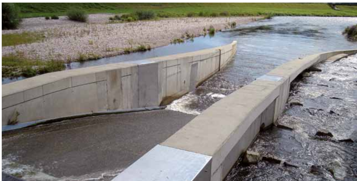
With the hydropower plant fish are free to pass above and below the turbine and various fish species have migrated through the river Kinzig to reach their former spawning grounds
