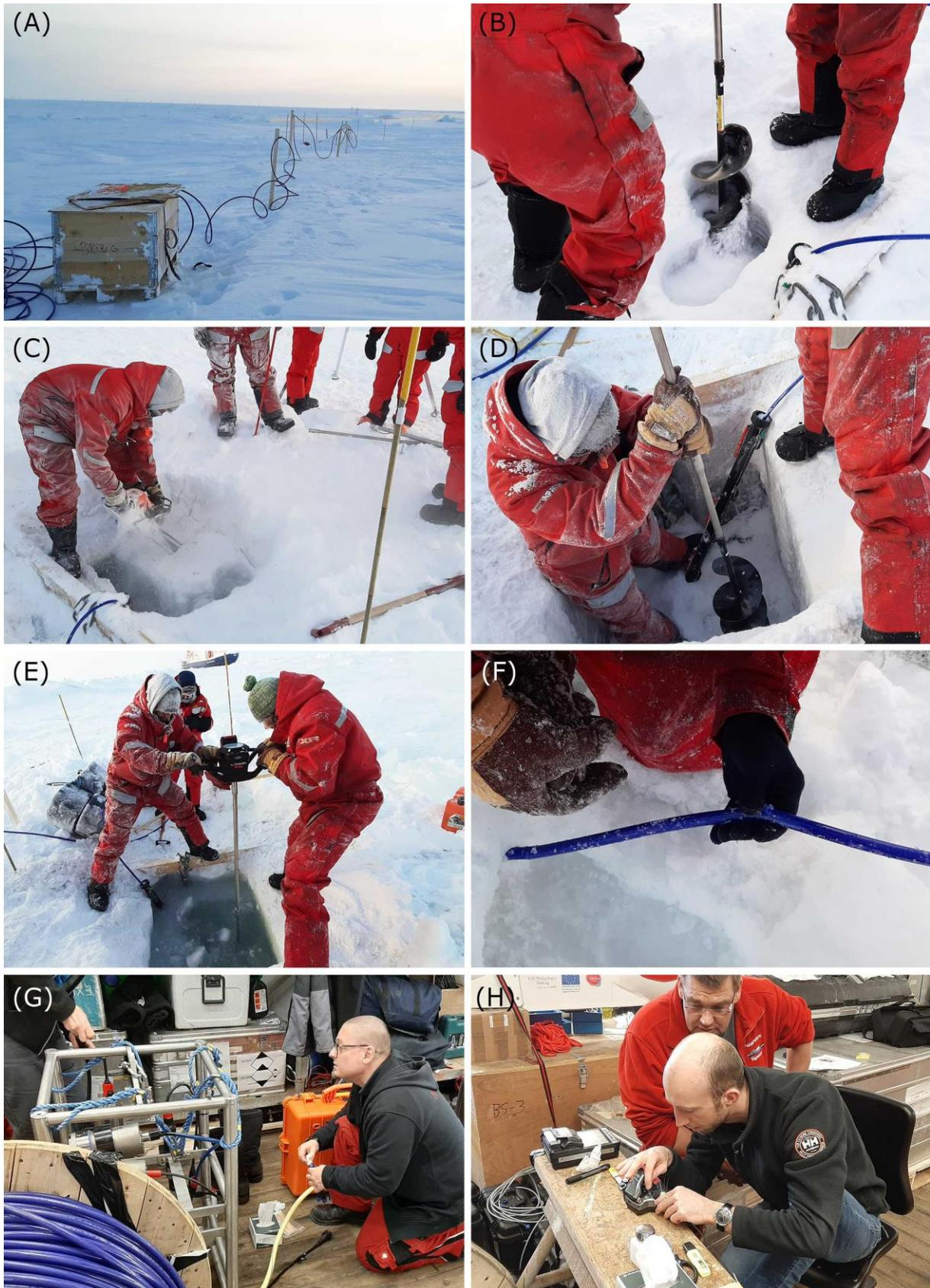
**Figure 35: Recovery and repair of the FishCam during Leg 3. (A) FishCam deployment site. (B,C,D,E) Recovery with the help of chain saw and auger, an operation that took two days on 17-18 March. (F) The broken cable. (G,H) Repair on-board by the *Polarstern* technicians. © Serdar Sakinan (A-H), 2020**
