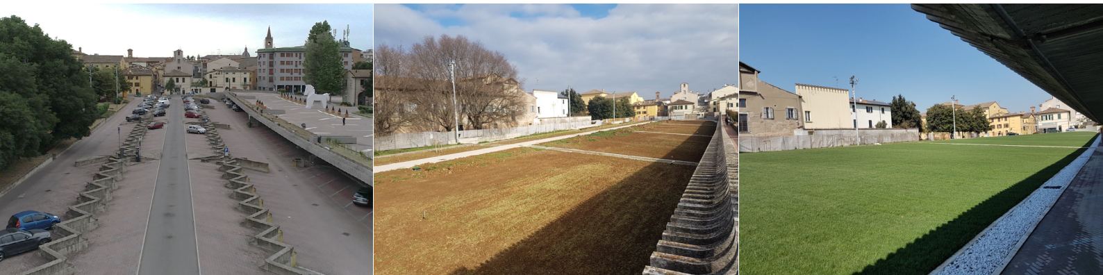
Figure 5. Demo site in Forlì (IT) before, during and after the de-sealing intervention
