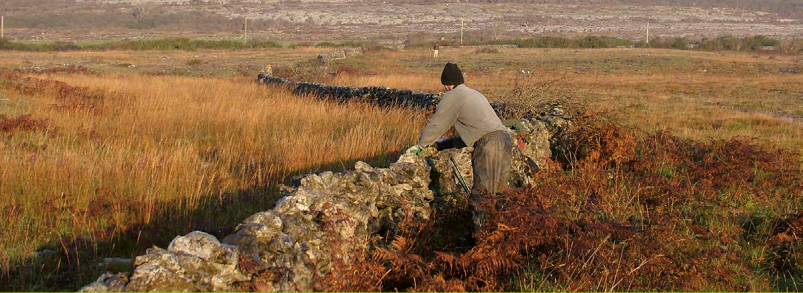
Photo: Repairing internal field walls to control grazing - LIFE04 NAT/IE/000125 - © EC
