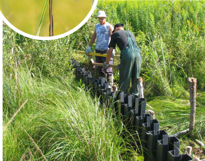
Photo: Blocking Amalva bog ditches with plastic piling - LIFE07 NAT/LT/000530 - © EC
