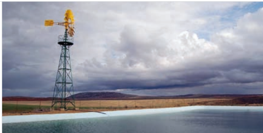
Cutting-edge technologies were combined to develop a simple and cost-effective method for minimising water use.
