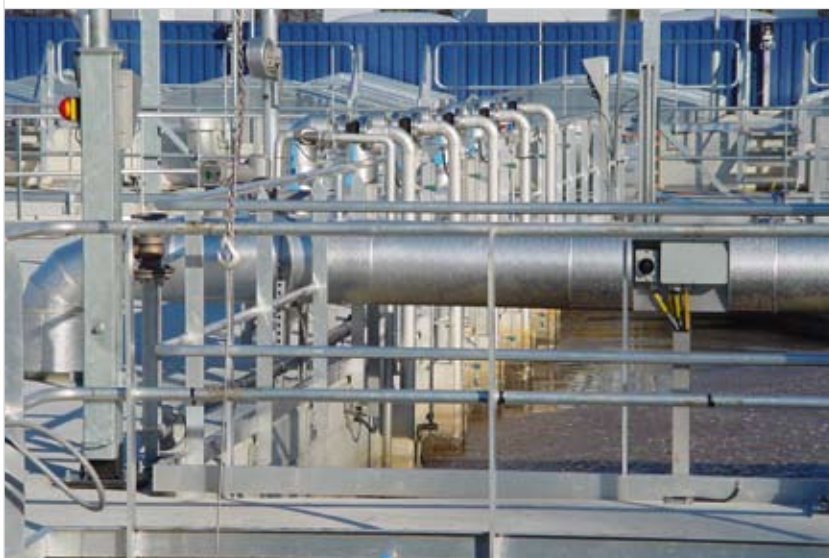
In the membrane tanks, water is separated from the bacteria-rich sludge by sucking it through membranes
