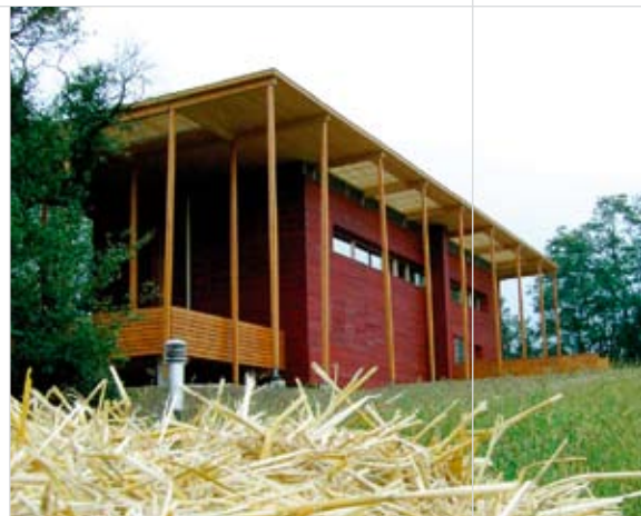
The S-House uses straw for its insulating properties
