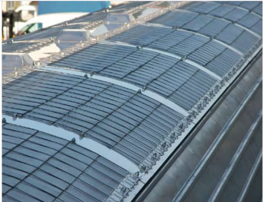
16 trays, curved with the same radius as the roof, carefully positioned
