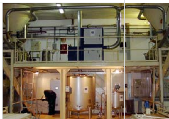
VPBs biodegrade VOCs into water and carbon dioxide
