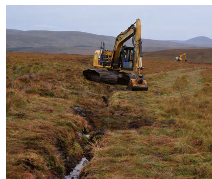
An excavator closing drainage ditches at the project site.
