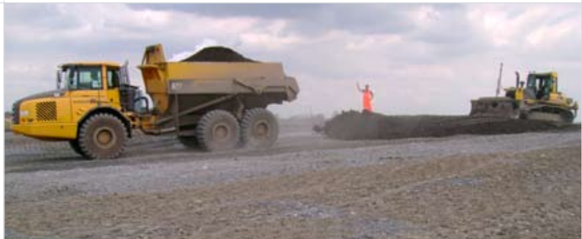
The project introduced an efficient surface sealing system for landfills that reduces use of natural resources (e.g. soil) and the dispersion of pollutants (e.g. sewage waste) in natural surroundings
