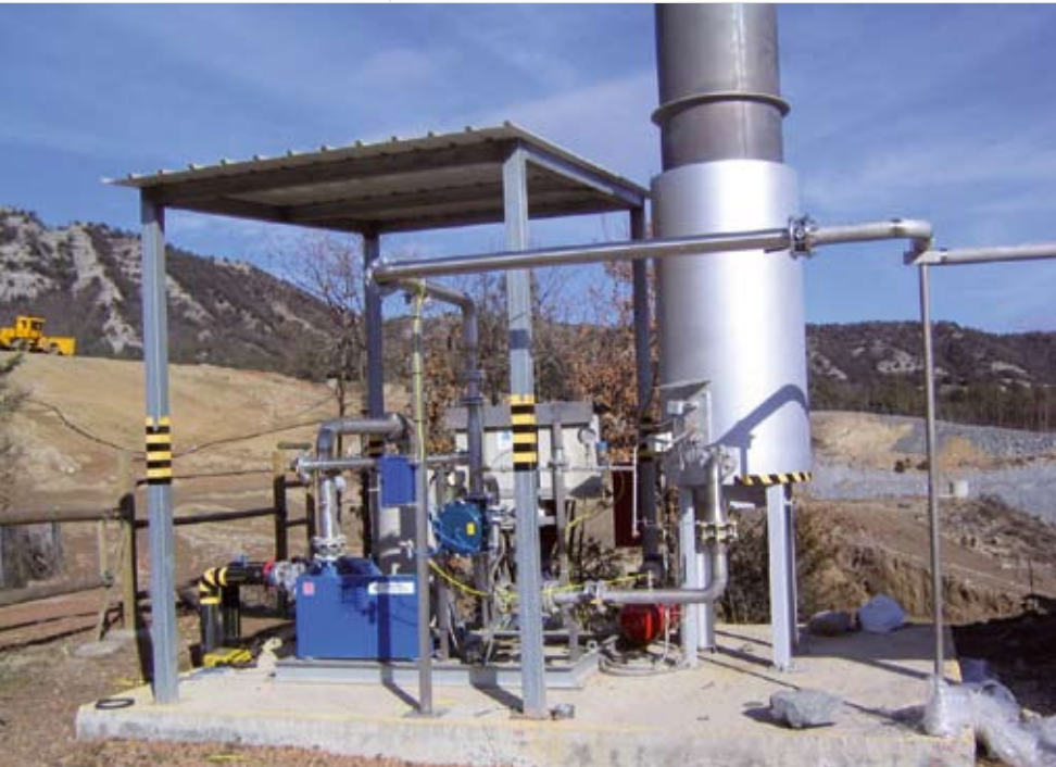
The MICROPHILOX project sought to demonstrate the first microturbine in Spain using biogas from a landfill in Orís
