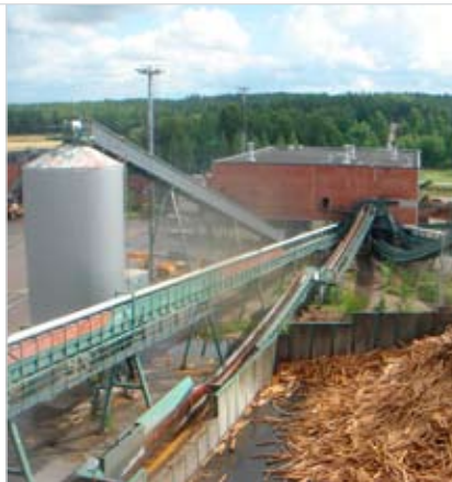
The project analysed selected airborne VOC emissions from different pulping processes and tested VOC abatement technologies, namely a catalytic incinerator plant in Finland and a biofilter-based pilot plant in Italy
