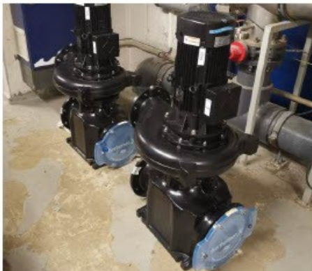
The new swimming pool circulation pumps
