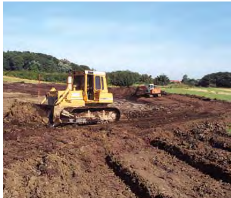
The project dug new ponds to enhance species connectivity
