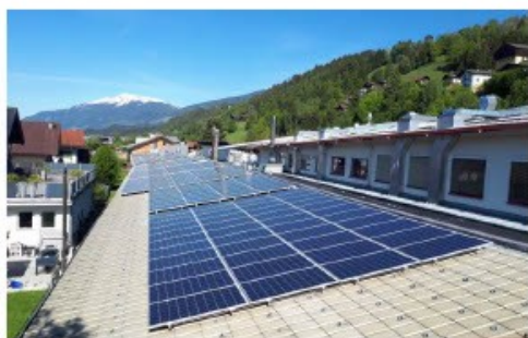
The newly installed 600 m 2 PV system covers 20% of Fahnen-Gärtner's electricity consumption
