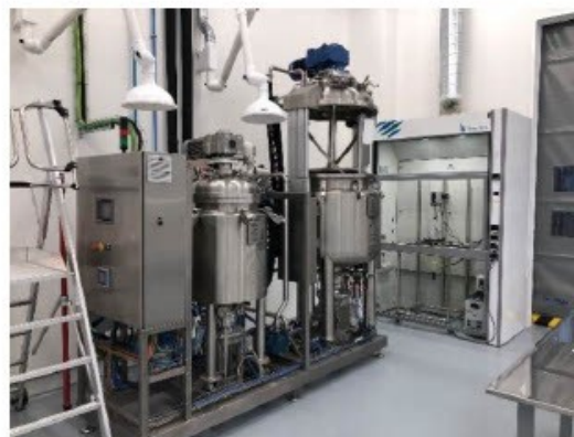
New encapsulation production line installed by Carinsa
