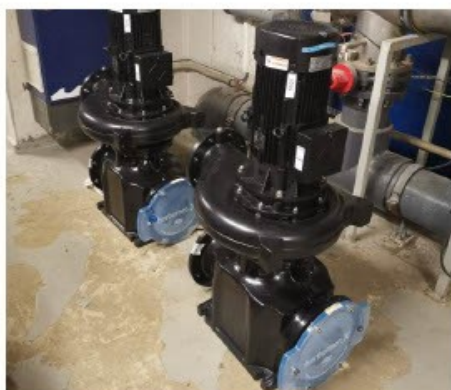
The new swimming pool circulation pumps
